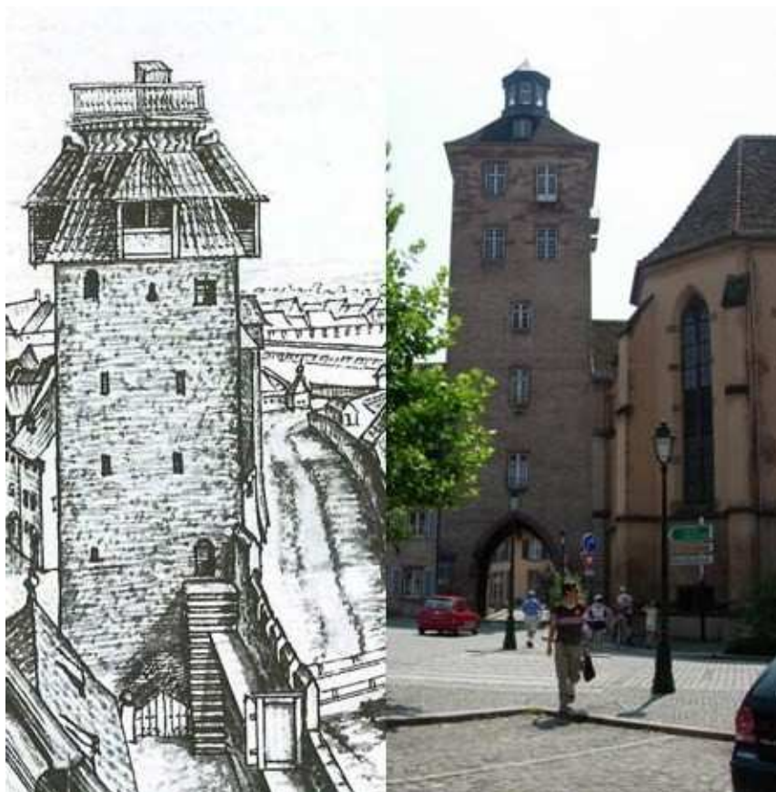
Figure 1. The top of Strasbourg Hospital Gate before its covering by a lantern (1671 pen-and-ink sketch by Johann Jacob Arhardt) and nowadays (© Cabinet des Estampes, reproduced with permission, & A. Heck). The structure visible on the ancient terrace is likely a shelter. The motivations recorded in the archives for the turret lantern were the prestige of the city and the notoriety of the university.
