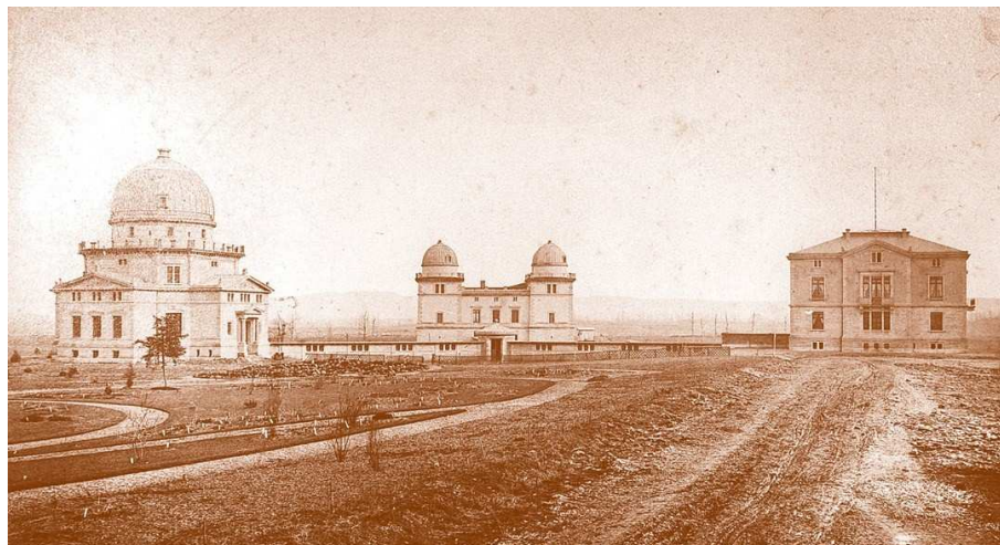
Figure 3. View around 1880 of the Kaiserliche Universitäts-Sternwarte Straßburg , the Wilhelminian observatory, showing (left) the dome of the Large Refractor, (center) the two smaller domes on a building housing also two meridian rooms, and (right) the Director's residence. The covered corridors linking the buildings are also visible. A few paths and young trees of the Botanic Garden are visible in the left foreground. The traces left by cartwheels on the right mark the future Universitätsstraße . The Imperial University including this observatory was the result of a deliberate political will from Berlin to have in Strasbourg a strong educational outpost. (Courtesy Strasbourg Obs.)
